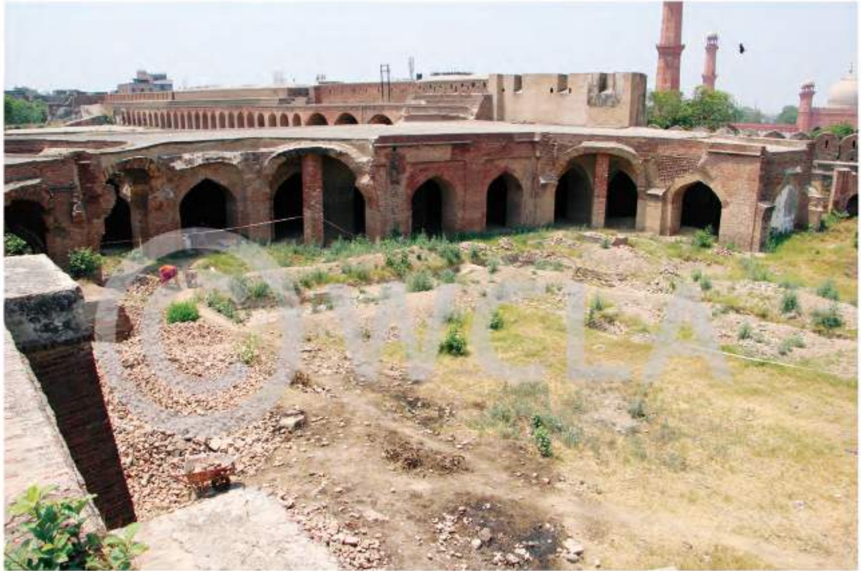
The image shows the cleaning of Royal Kitchens before Restoration
